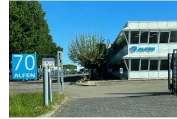
Battery Factory Damsluisweg 70
